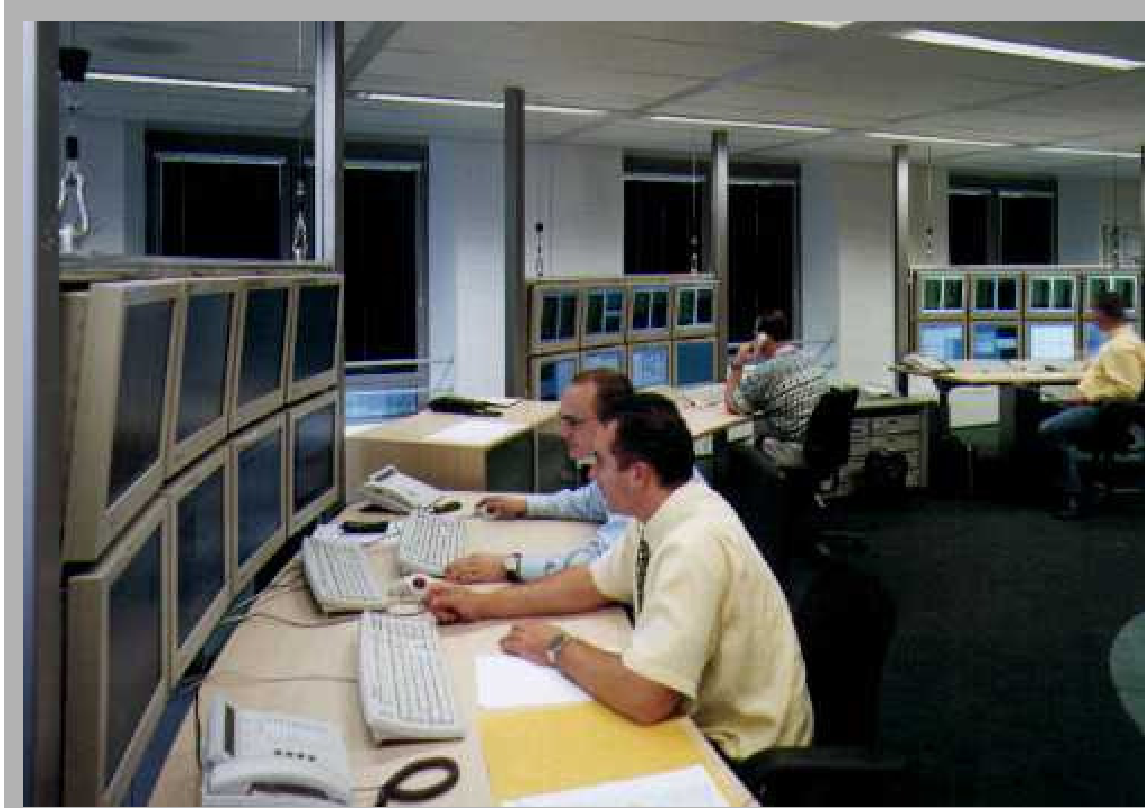
Network Control Center : Vodafone (The Netherlands)
